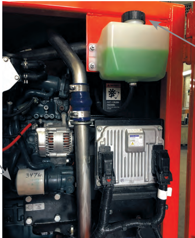
Check coolant level
